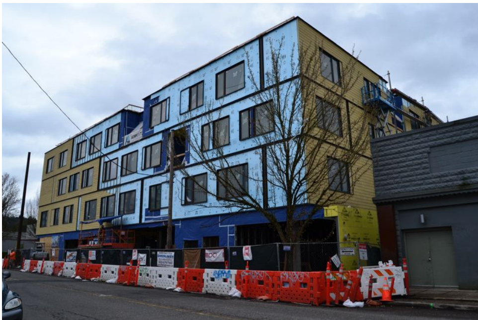
PAMPLIN MEDIA GROUP: JULES ROGERS - Siding is being installed on the cohousing project now, which will also include solar panels, a rooftop garden, a commercial kitchen and large interior common areas.
